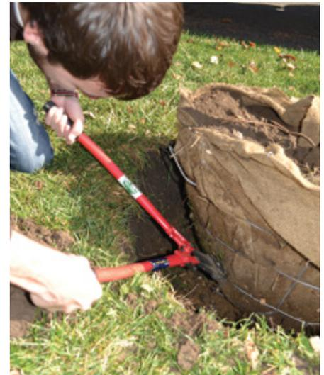
*Using wire or bolt cutters, remove all or at least the top portion of the wire basket to prevent interference with roots as the tree grows.*
